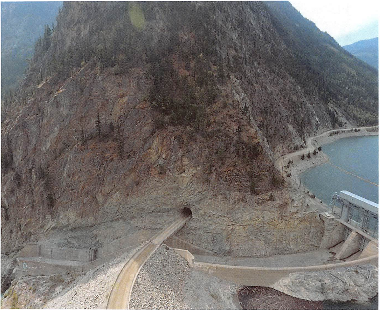
Terzhagi Dam with Highway 40 crossing the Spillway.
