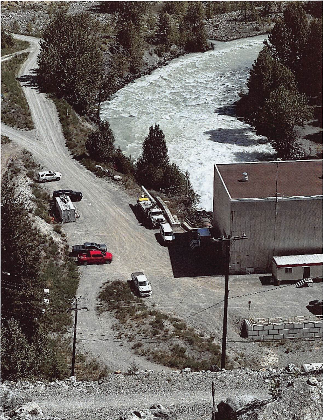
Powerhouse and Bridge River from the crest of the LaJoie dam
